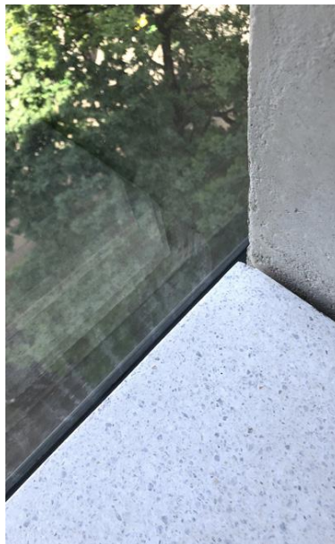
Window detail in the open circulation space. Photo by author (2022).
